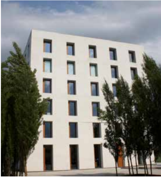
Figure 1: Haus 2226, Baumschlager Eberle. Source: (Author 2016)
