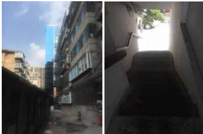
Fig. 5: An investigated dwelling which was added an elevator this year.
