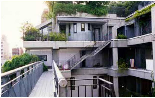
Yoshitka Utida /Shu-Koh-Sha Architectural and Urban Design Studio, NEXT21, Osaka, Japan, 1993- present
