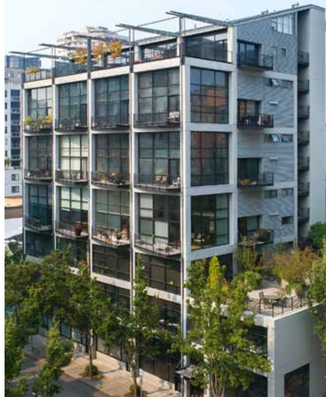
The Banner Building, Seattle, WA; Weinstein AU Architects + Urban Designers LLC
