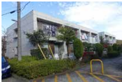
Figure 4: The terrace house Source: (Author 2017)
