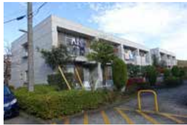
Figure 4: The terrace house Source: (Author 2017)
