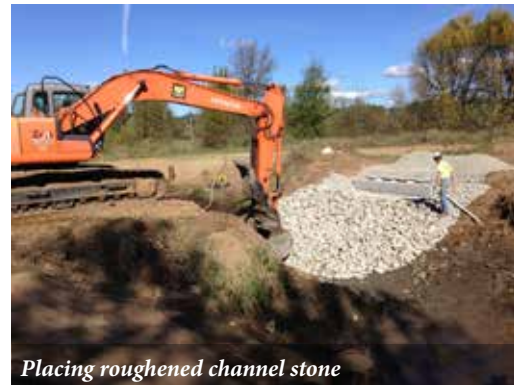
After: crossing and roughened channel installation
