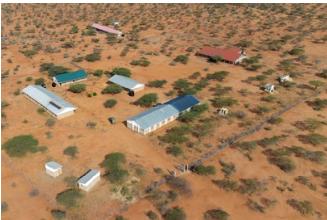
Fenced Lenkuruma Primary School to enhance safety within the school compound.
