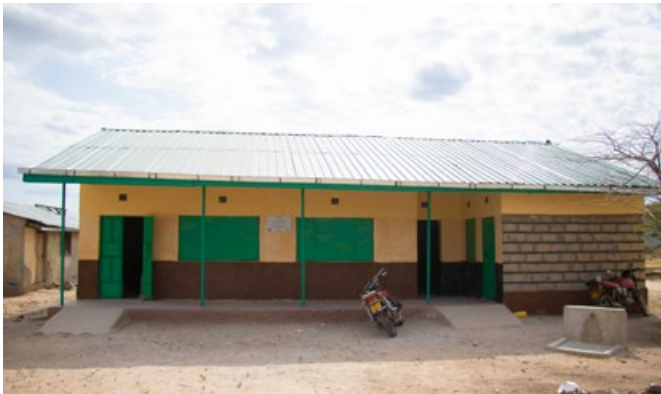
Constructed Goda Primary School's administration block.
