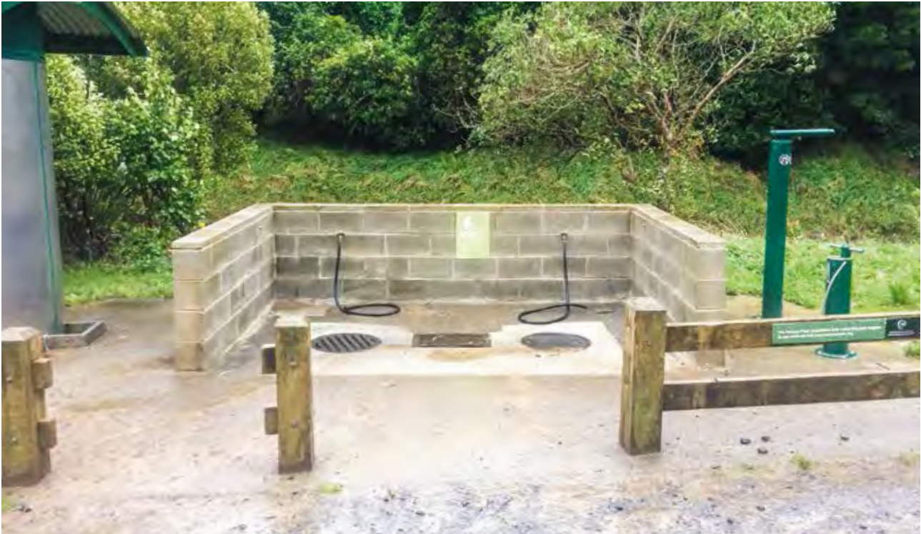
Figure 6: Existing bike wash and maintenance facilities at main car park.
