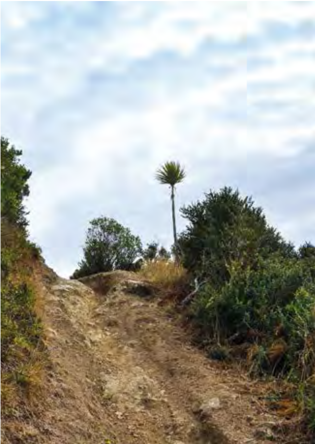
Figure 5: Ongoing wear and scour on upper sections of Ridge Line track.
