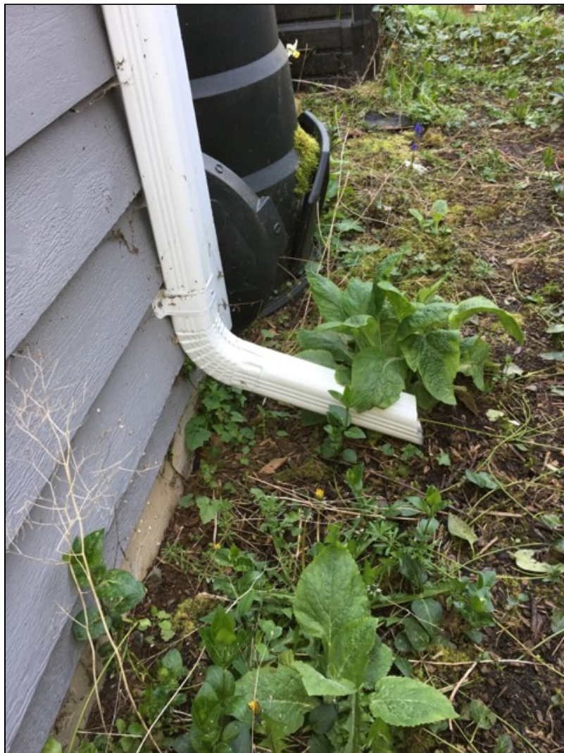
2.1 Item 1(Picture) Downspout at side of house
