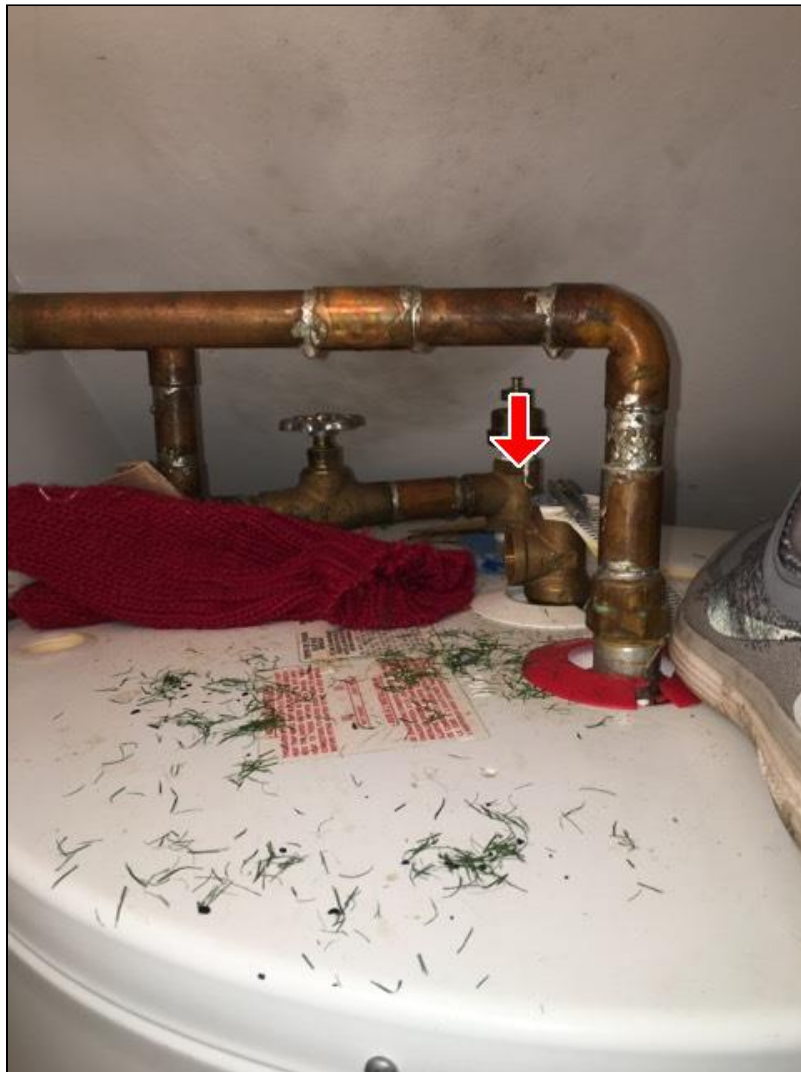
7.4 Item 1(Picture) Drain tube required for T and P valve
