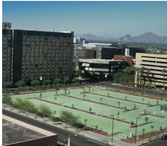
*Figure 3.12. Reflective pavement on a parking lot<sup>51</sup>*
