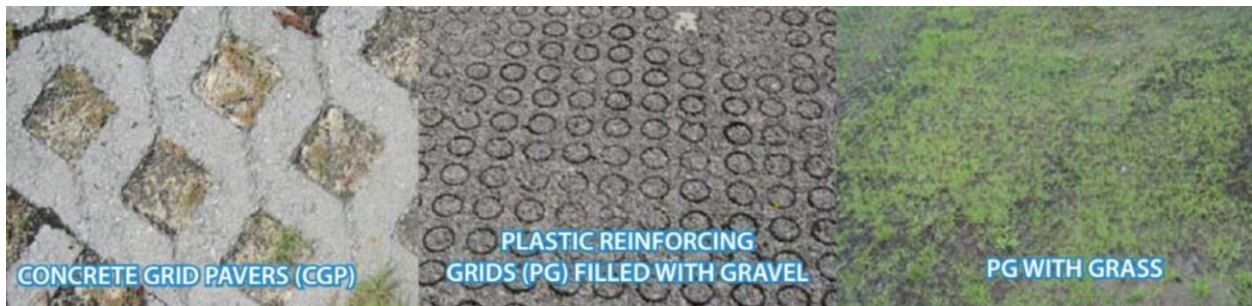
Figure 9.39. Examples of grid pavements. 412
