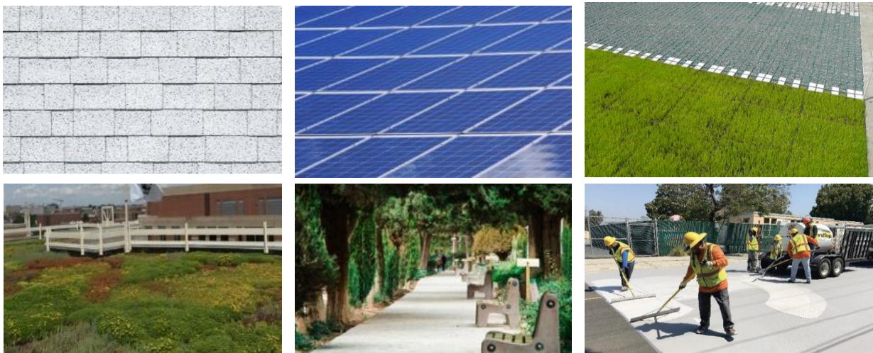
Figure 4.1. Images of Smart Surfaces (from left to right and top to bottom: cool roofs, solar PV, permeable pavements, green roofs, urban trees, and reflective pavements)
