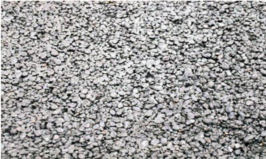
Figure 7.9. Example of a porous pavement with a higher albedo.
