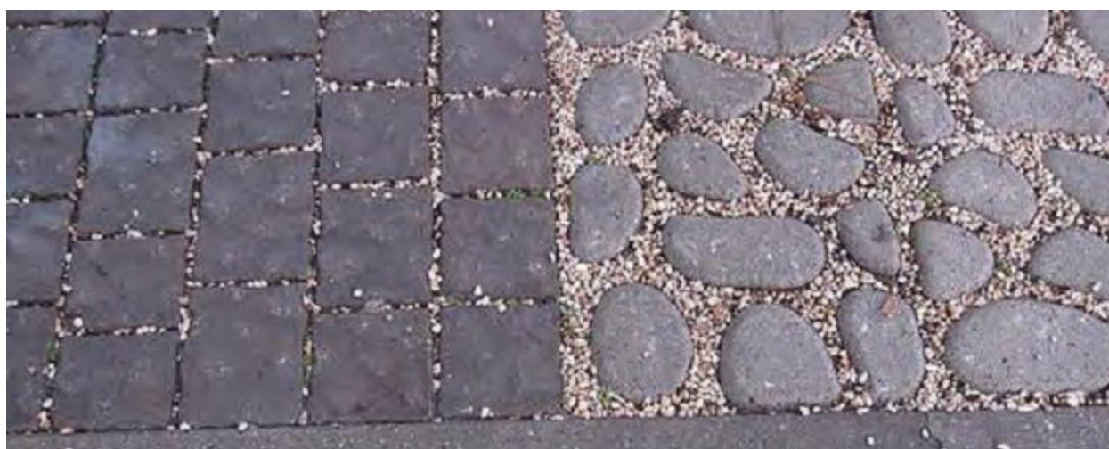
Figure 9.38. Examples of permeable pavers. 409
