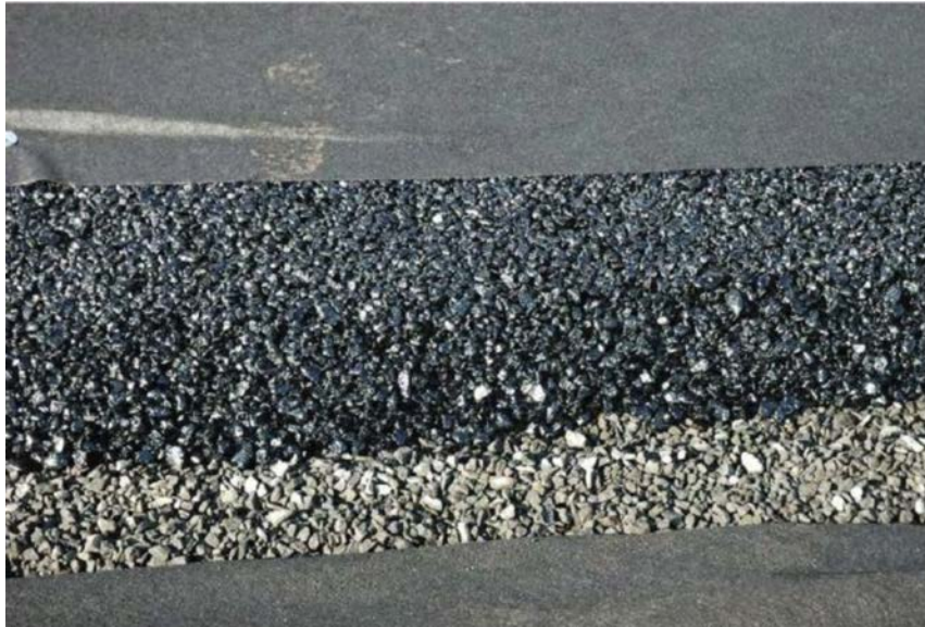
Figure 9.36. Example of porous asphalt pavement. 400
