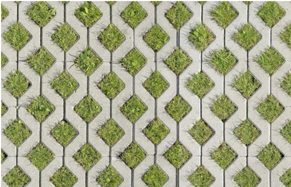
Figure 7.10. Example of a green, porous parking lot pavement.
