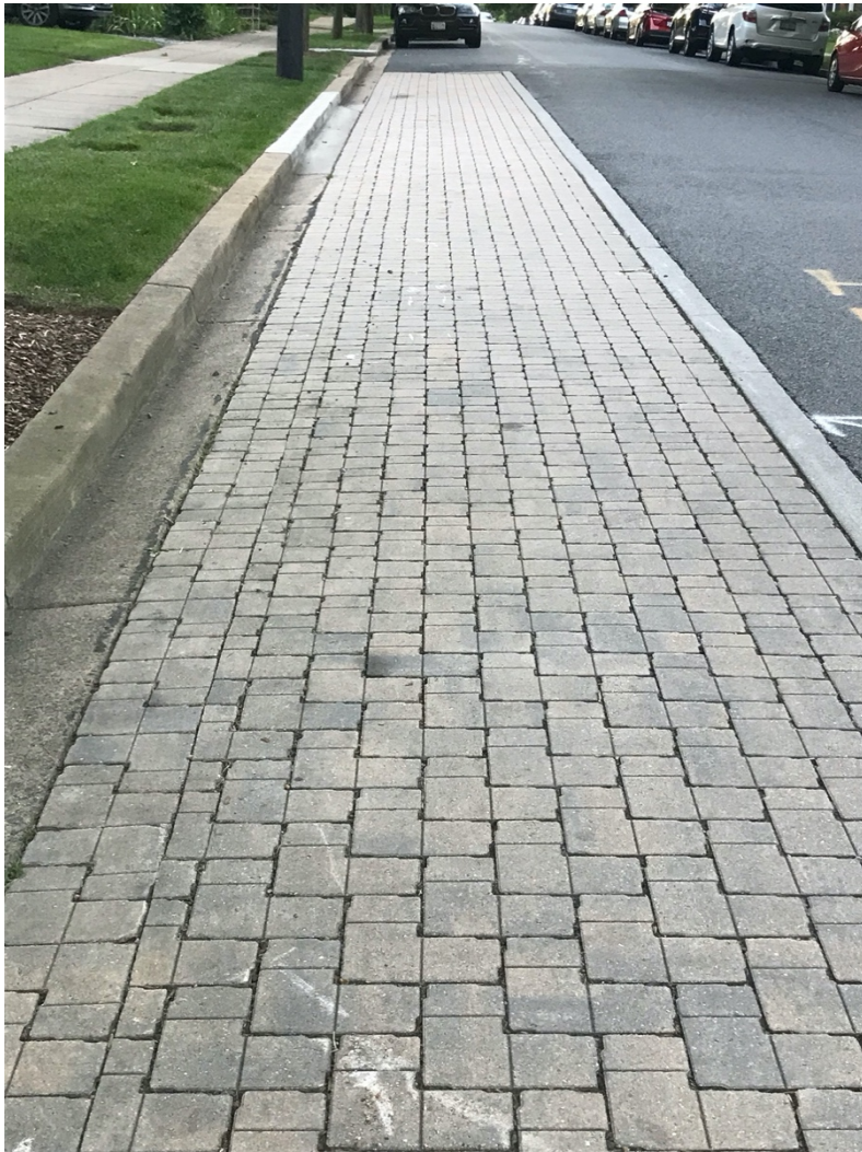
Figure 7.8. Example of a reflective pavement with a higher albedo than conventional pavement.
