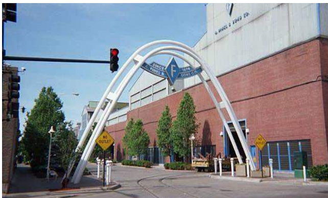
Example of an industrial entry arch
