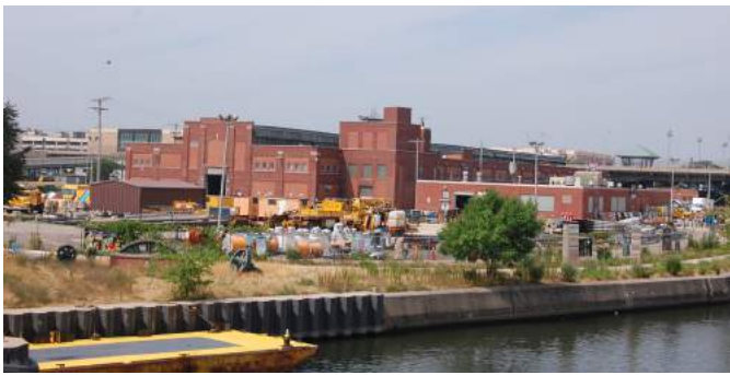
The Milwaukee Dept. of Public Works vehicle yard adjacent to the Menomonee River
