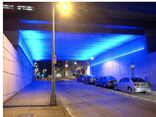
Decorative LED lighting provides aesthetics & pedestrian comfort to highway overpass
