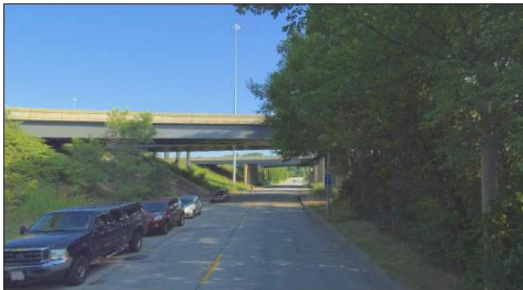
An improved N 44th St. can provide a key bike and pedestrian linkages between west side neighborhoods and the Valley
