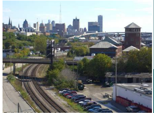
Rail and Viaduct Infrastructure
