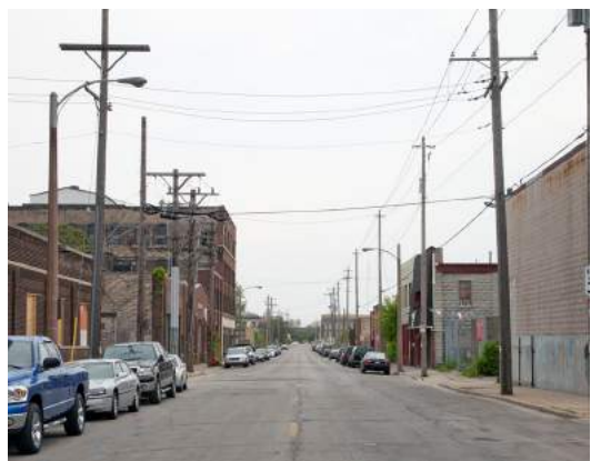
View of W Pierce St. looking east Source: Dept. of City Development
