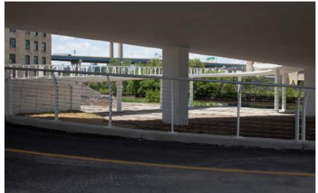
Bicycle access between Walker's Point, The Tannery, and Reed Street Yards with 6th St. Viaduct
