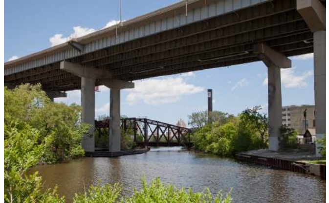
Train bridge over the Burnham Canal Source: Dept. of City Development
