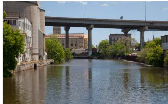
Burnham Canal looking east Source: Dept. of City Development
