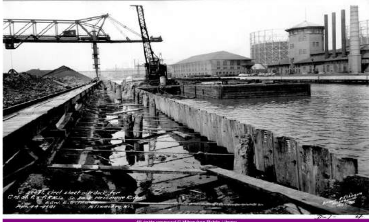
Menomonee River Dockwall Construction, Circa 1941
