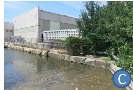
Milwaukee Recycles Building and truck traffic / storage <25' from water edge
