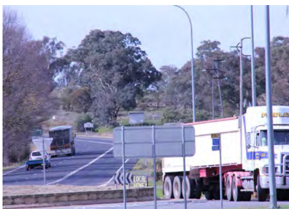
The Roundabout at Wallendbeen
