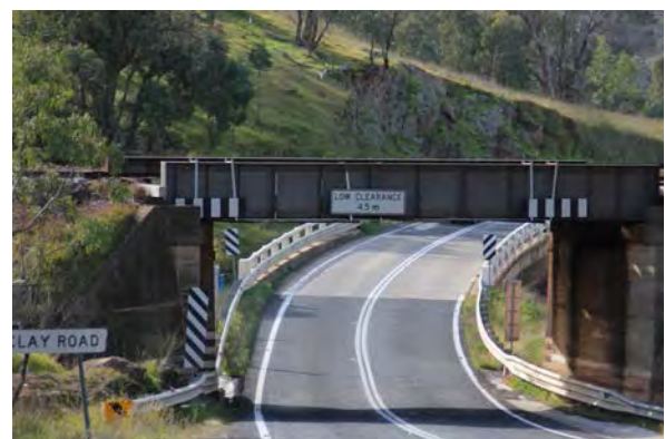
The Gap Bridge, Olympic Highway at Cootamundra
