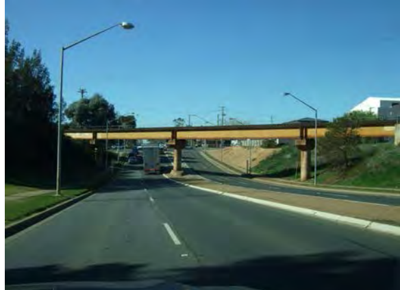
The rail-over-road bridge on the Sturt Highway at Wagga Wagga
