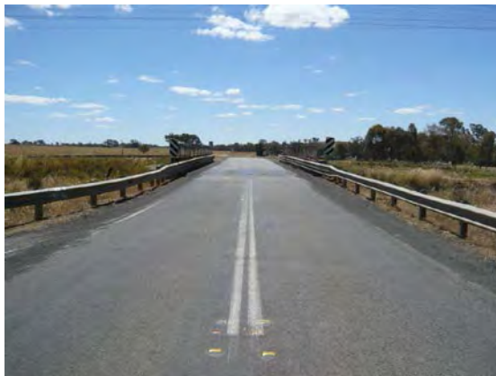
Causeways on the Burley Griffin Way are subject to flooding
