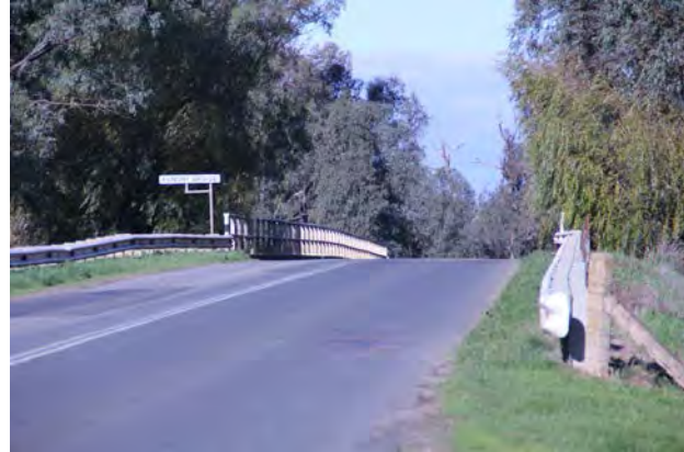
Eunony Bridge at Wagga Wagga
