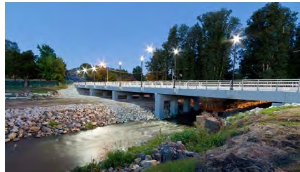
New bridge constructed over the Adelong Creek at Adelong, opened February 2011. (photo: NSW RTA)
