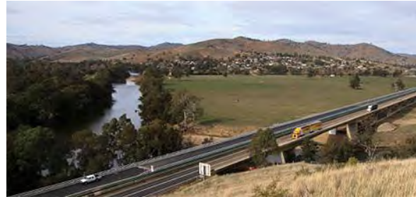
Sheahan Bridge at Gundagai is not approved for A-Doubles (photo NSW RMS)
