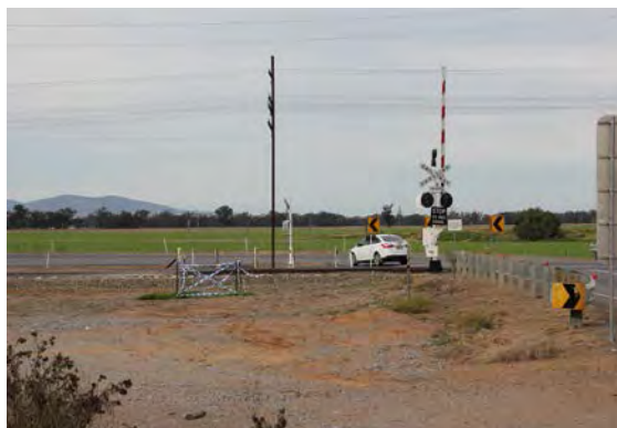
Right angled bend on the Main Southern Rail line north of Illabo
