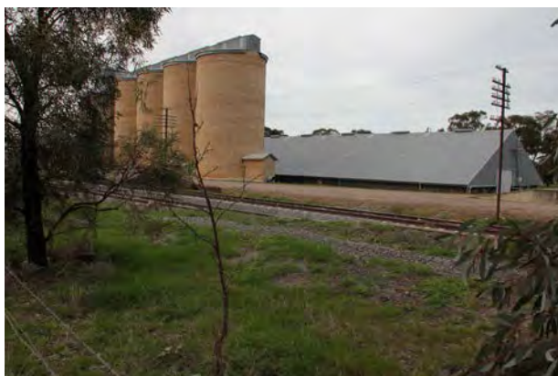
Major grain receival facility located on the Main Southern Rail Line at Illabo in Junee Shire
