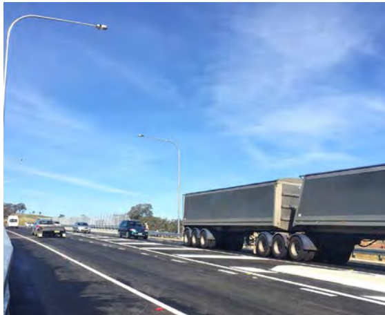
The new Kapooka Bridge was opened in July 2016
