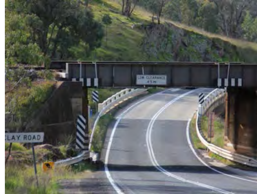
Suttons Lane is the high vehicle detour for the Gap Bridge (pictured) at Cootamundra
