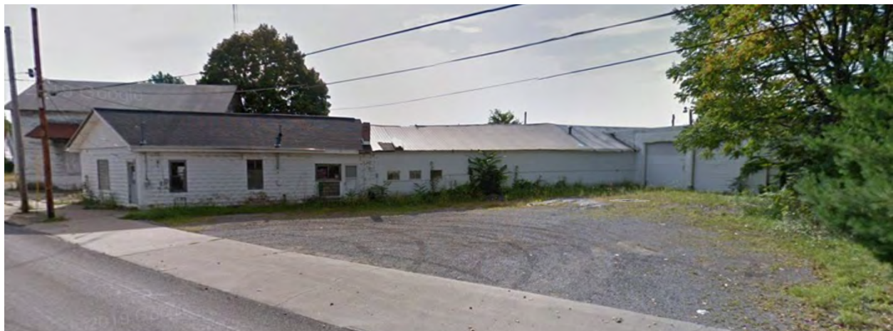
View from Clinton St looking northeast
