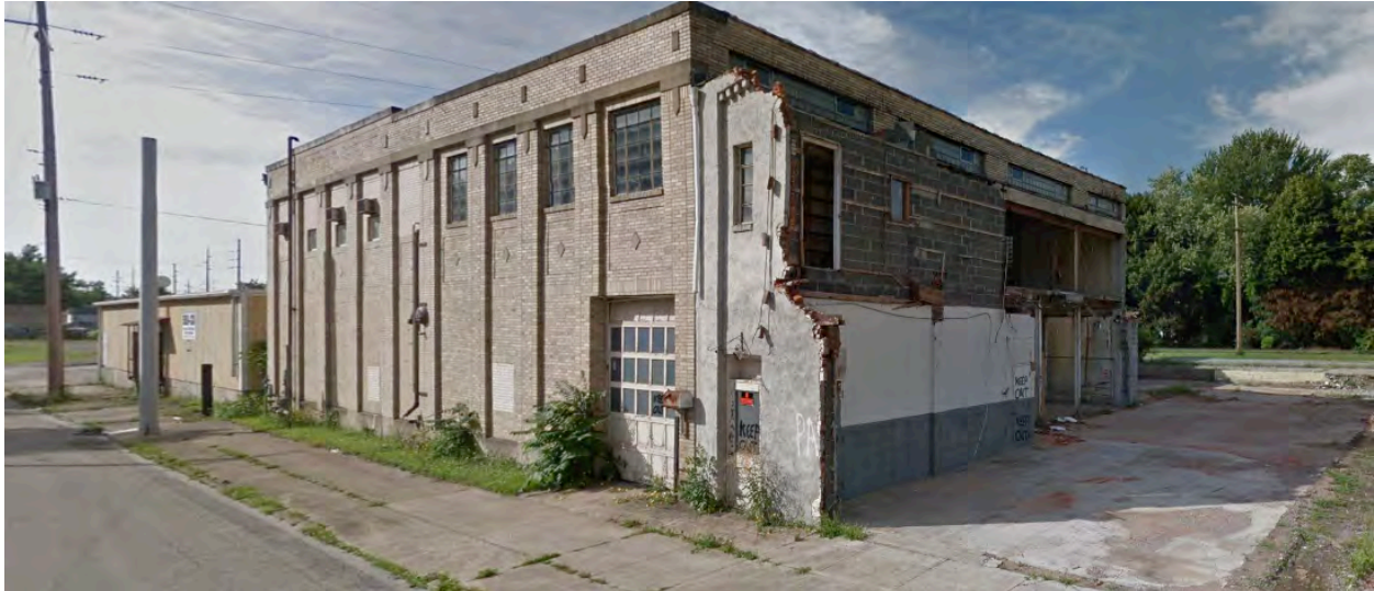
View looking south along Canal St
