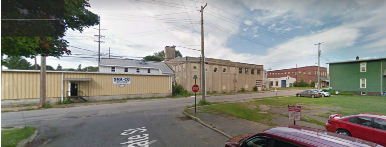
View looking west from Canal St. and State St.
