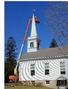
Painters working on the steeple.
