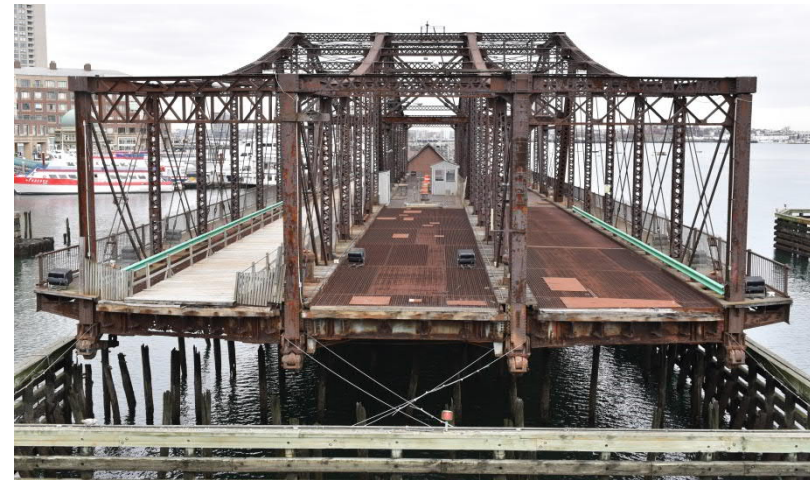
Existing Northern Avenue Bridge
