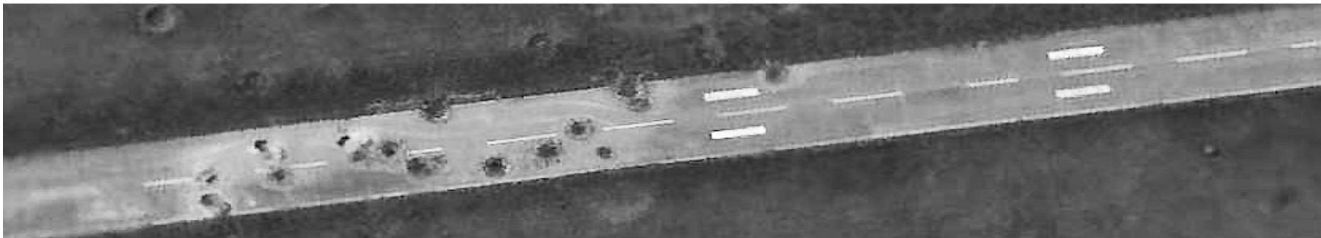
Figure 3: Runway damage following a denial attack.
