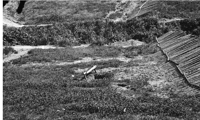
Civil War era photo of a sink or latrine (photo middle) consisting of a dug hole in the ground with single log and supports.
