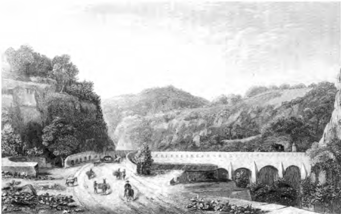
Stone bridge constructed in 1806 near Veracruz
