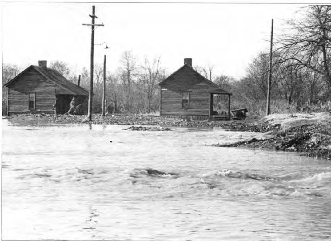
Two Negro tenements on North Margin and 2nd Ave. North during the Flood of 1948.
