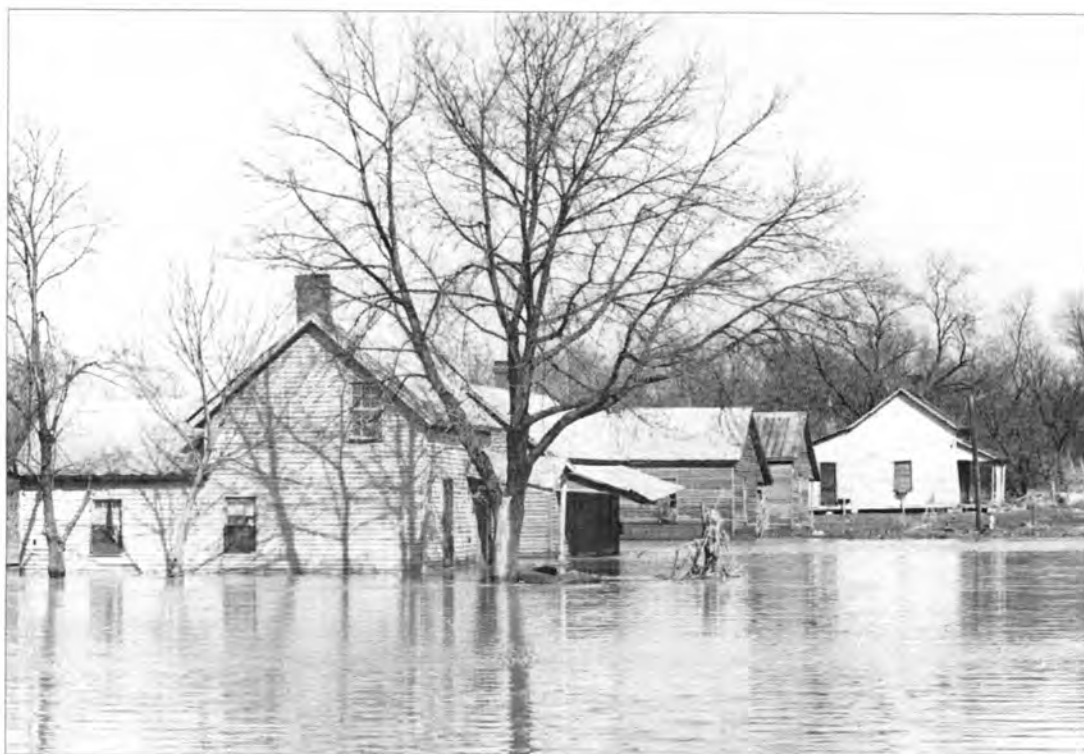
Eggleston's Bottom on North Margin Street during the Flood of 1948.
