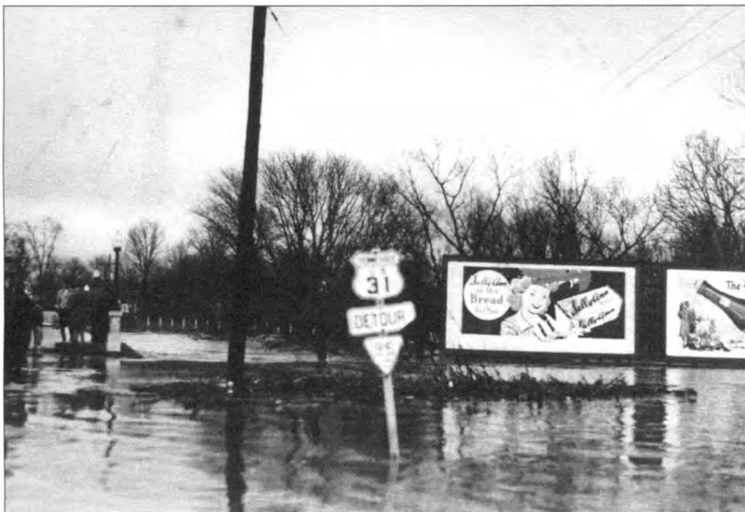
At the Nashville Pike Bridge on East Main Street during the Flood of 1948.
