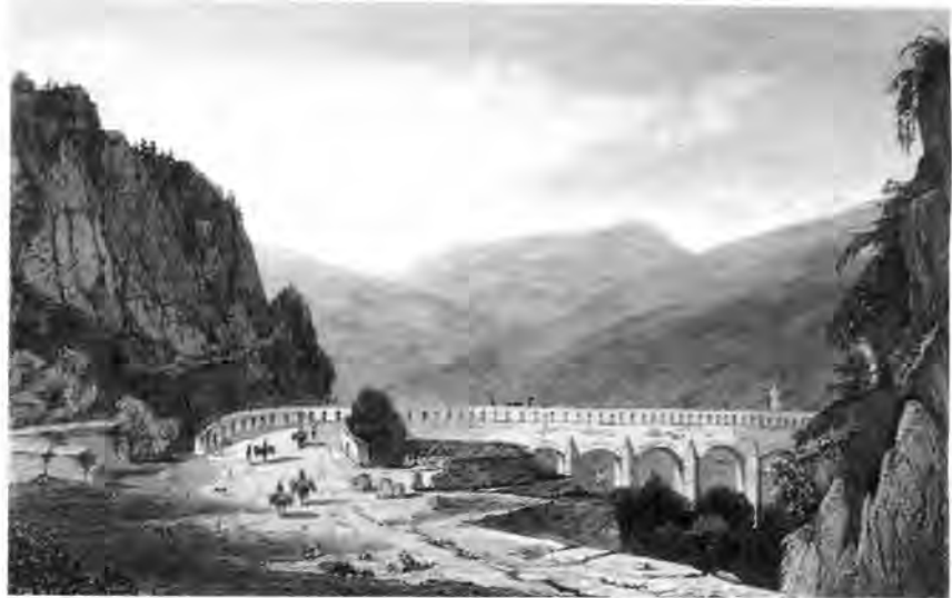
Stone Bridge constructed in 1806 near Veracruz
