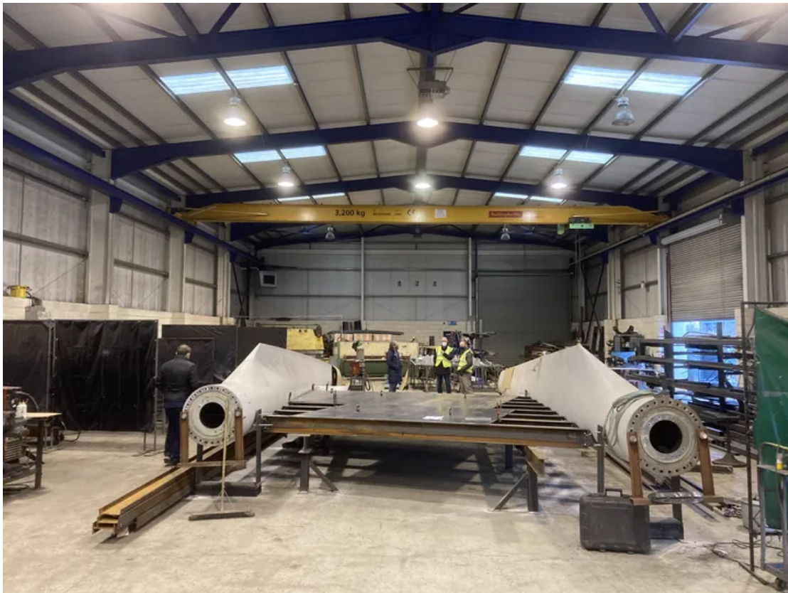
The ReWind bridge's first blade bridge was test assembled before being installed along a new pedestrian greenway. | ReWind
