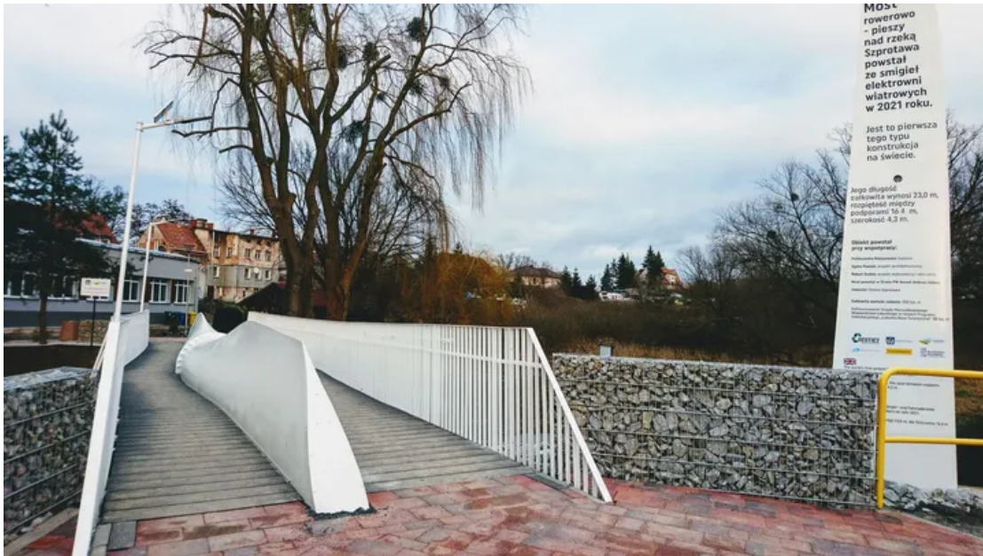
The world's first wind turbine blade bridge was recently installed in western Poland. | Anmet
