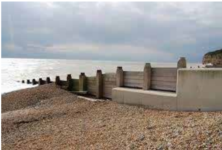
Concrete & wooden Groyne, Pett Levels cc-by-sa/2.0 - © N Chadwick - geograph.org.uk/p/1503224
