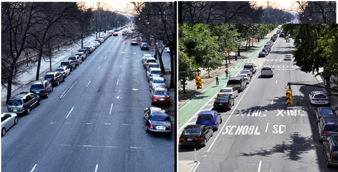
The insertion of a cycle track on this Brooklyn street dramatically improved safety for all road users without reducing daily car through-put.
