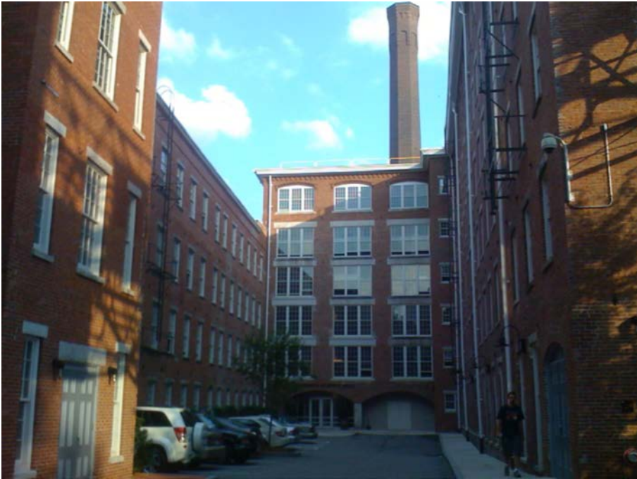
Lowell, MA almost doubled its downtown housing stock from 2000 – 2011, largely through historic rehabilitation.
