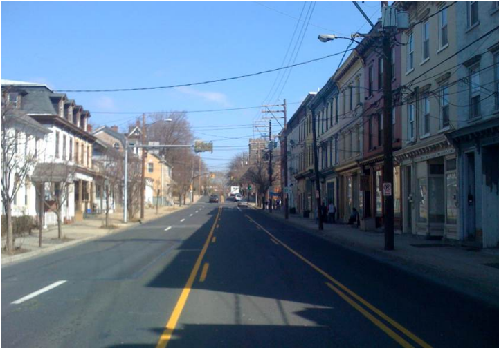
In Bethlehem, PA, an unnecessary and overlong turn lane has eliminated a block of curb parking, contributing to the failure of most adjacent businesses.
