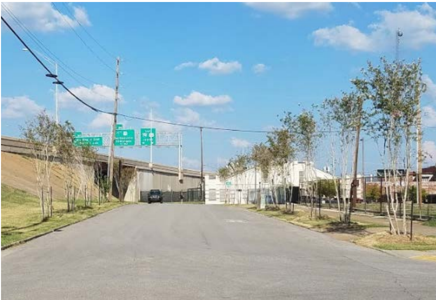
Crepe myrtles, like those planted along Easton Street, provide little shade while crowding adjacent sidewalks.
