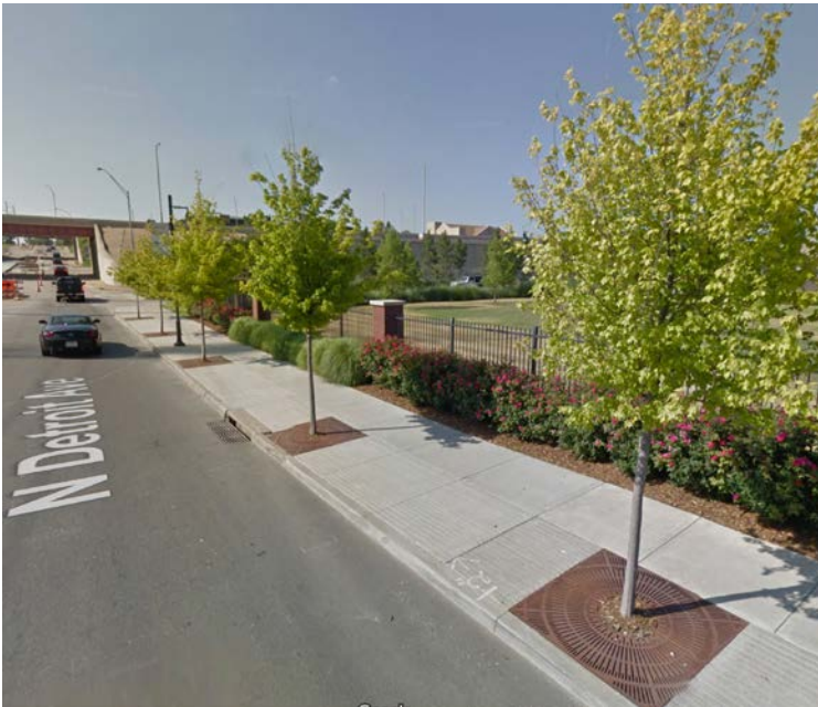
New sidewalks on Detroit, MLK, and elsewhere suggest a proper tree-planting standard is in place.
