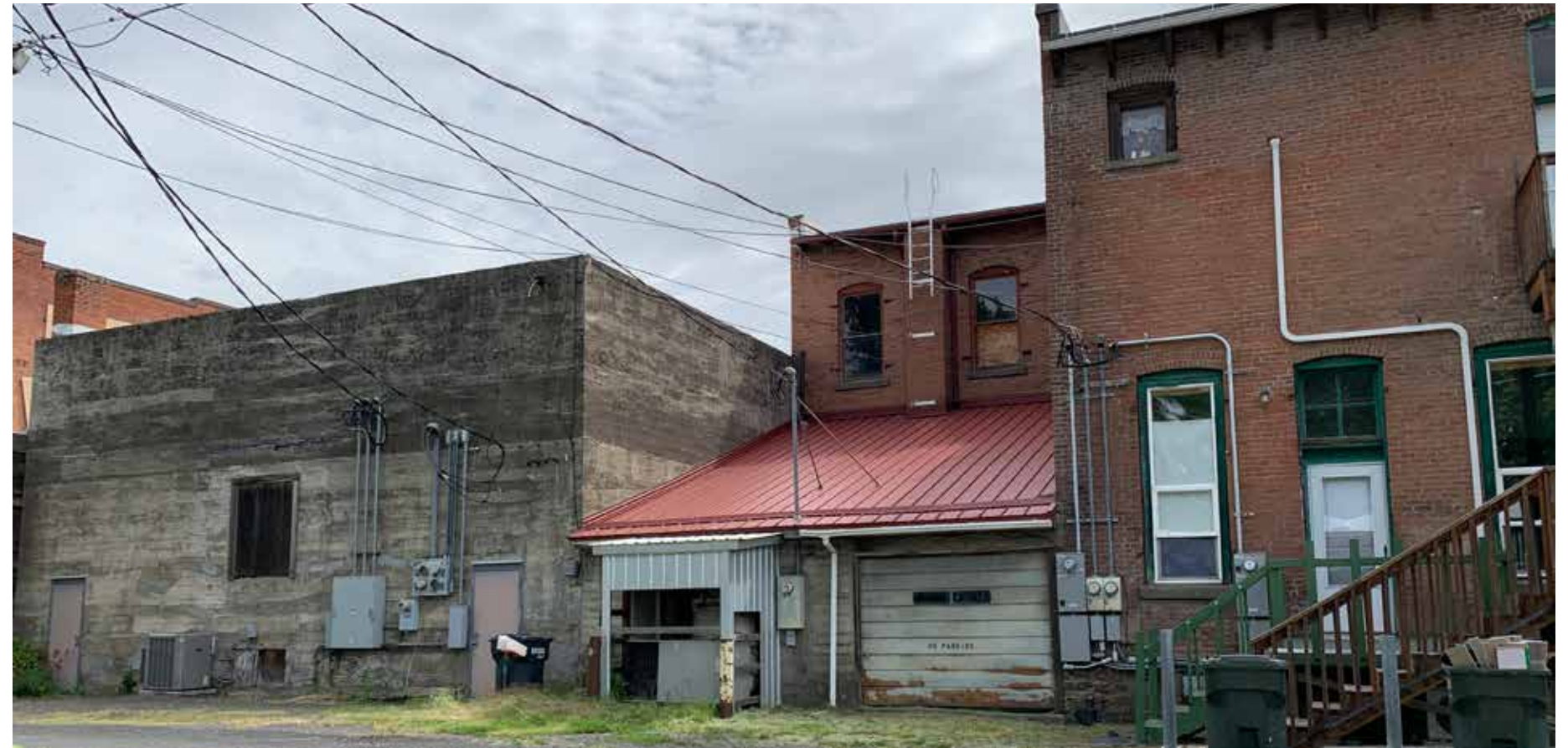
EXISTING WEST PATIO
