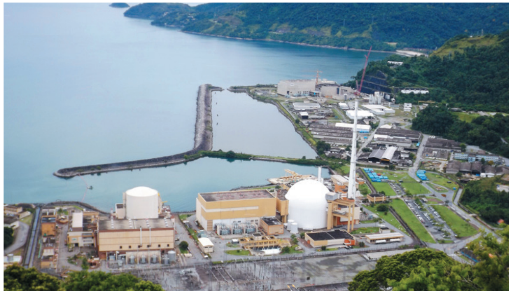
Angra Nuclear Power Station in 2017 (Photo by Divulgação PAC/Agência Brasil)
