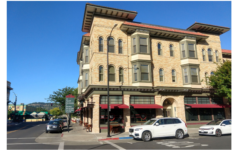
Example of a mixed use building in downtown Napa.
