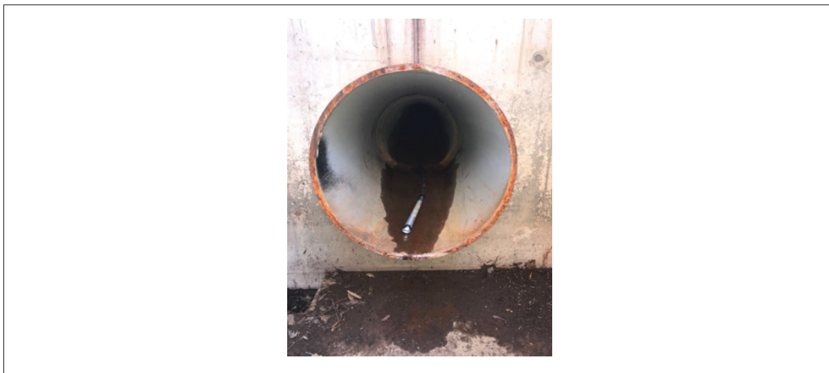
Figure 3.4: Hydrophone array in Pit 1 with battery pack attached. Array close to filled. Photo taken just prior to pipe section reinstalled at Pit 1 and test bed fully filled. 6.2
