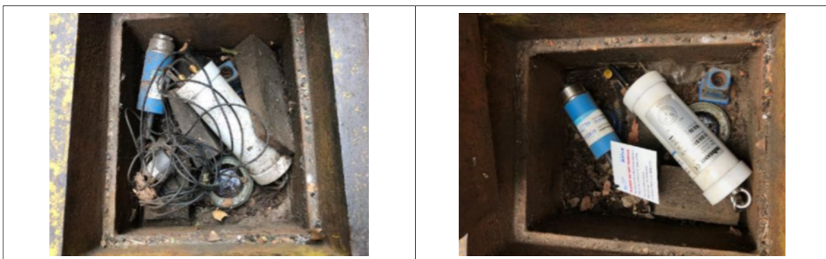
Figure 4.13: Seba Log N-3 Sydney CBD upgrade. GPS/GSM antenna left, GSM stubby antenna right.
