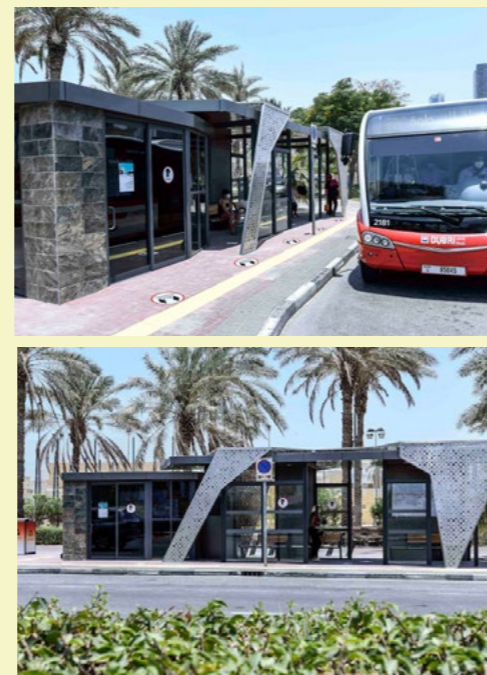
Figure 7: New bus shelters
