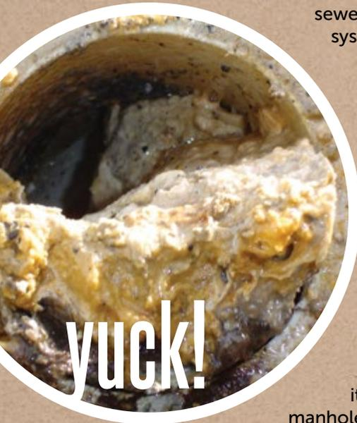
Grease is the most common cause of sanitary sewer overflows. When people cook and pour fats, oils, and grease (also known as FOG) down the drain, the FOG turns from a liquid to a solid as it cools, clogging the pipe. When the water can't make it past the greasy mess, the pipes back up. Sometimes it is so powerful it can push up a manhole and flow into the street. Once wastewater is on the street, it acts just like rainwater and flows to the storm drain.
