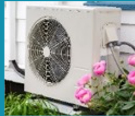
Air source heat pumps
