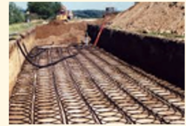
Ground source heat pumps
