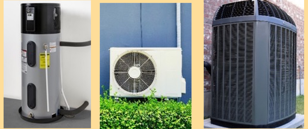
Heat pump technologies: Heat pump water heater, mini-split, ducted heat pump
