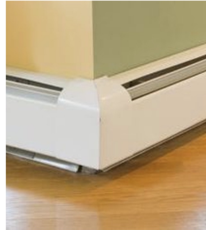
Electric Resistance ~100% efficient
