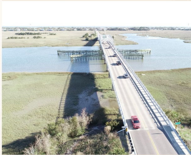
Ben Sawyer Bridge to Sullivan's Island/ Mount Pleasant
