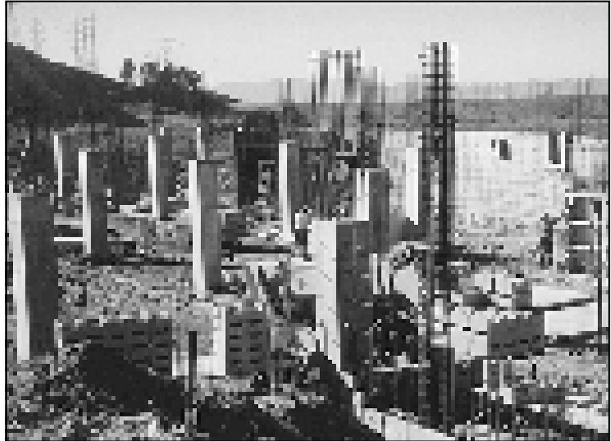
▲ *Emergency Vehicle Operations Center - Building #1 ground level formwork for vehicle storage area.*
