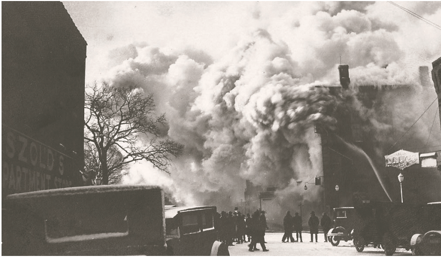
Image • The Academy of Music Block Fire rages at the southwest corner of Washington Street and Lincolnway, 1926.
