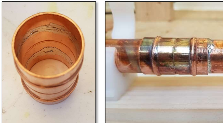
Figure 53: Solder fitting, before and after installation
