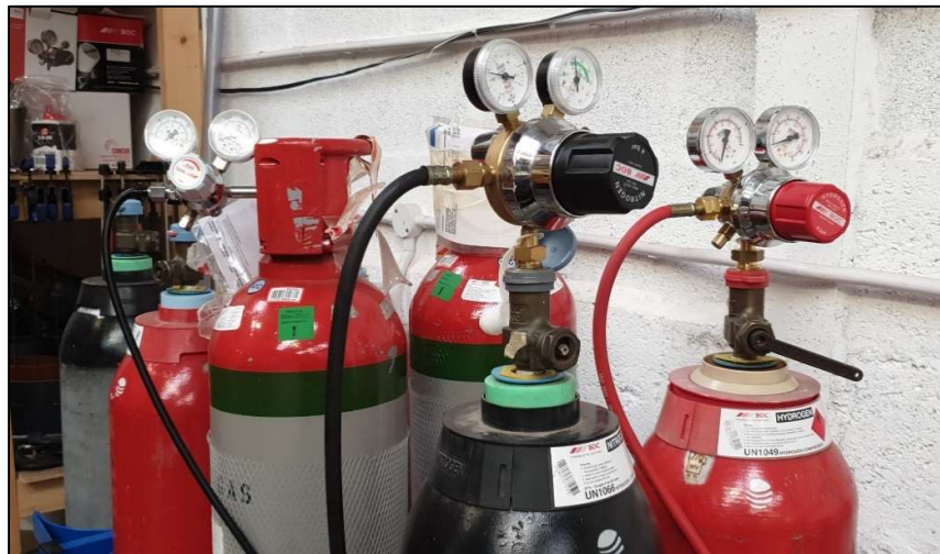
Figure 16: Gas cylinders with 4 bar regulators
