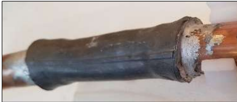
Figure 56: Sweated lead to copper
