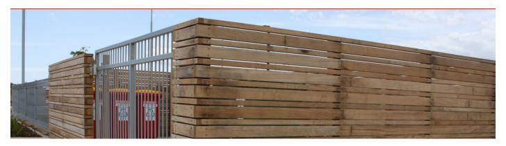
Horizontal slats provide great privacy screening as infill on block walls, gates and screening around services. Choose from privacy spacing with narrow 10mm gaps or airflow spacing with larger 16mm gaps.
