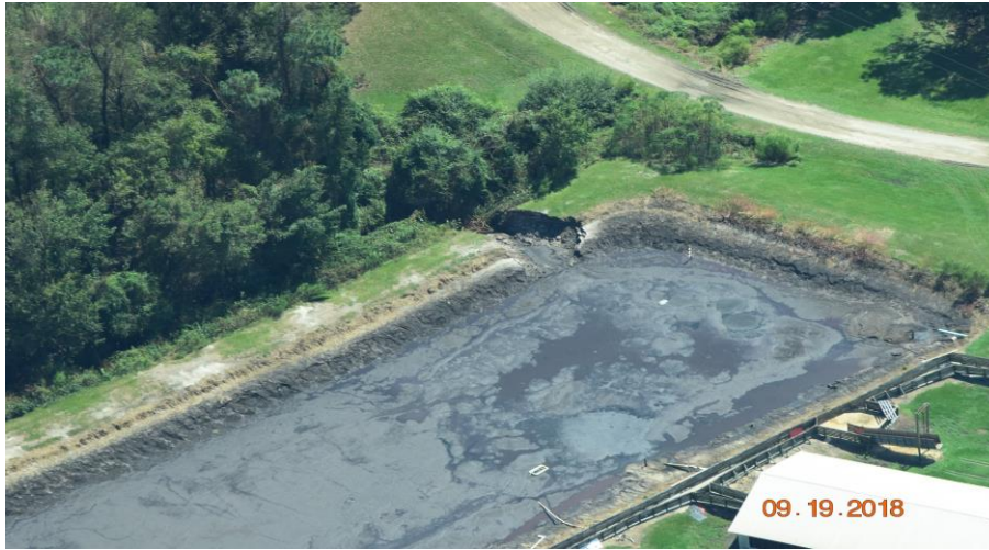
Hog lagoon breach near Stockinghead Creek in Duplin County days after Hurricane Florence. Photo courtesy of Waterkeeper Alliance, Inc.
