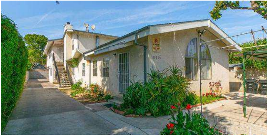
2 11315 Tiara St 11315 Tiara St North Hollywood, CA 91601
