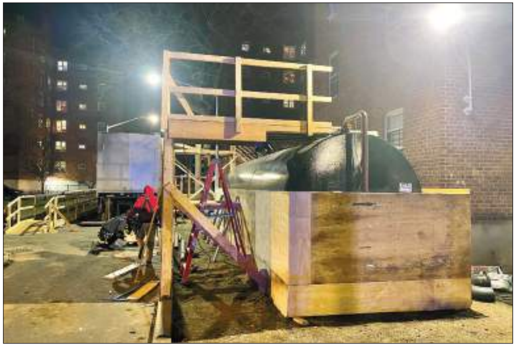
A bill that would adjust utility costs for NYCHA residents during outages moved forward in the State Senate. Several Queens NYCHA residencies have seen long-term utility outages recently, including a heat and hot water outage in the Woodside Houses that required the installation of mobile boilers, pictured here. Eagle file photo by Jacob Kaye
