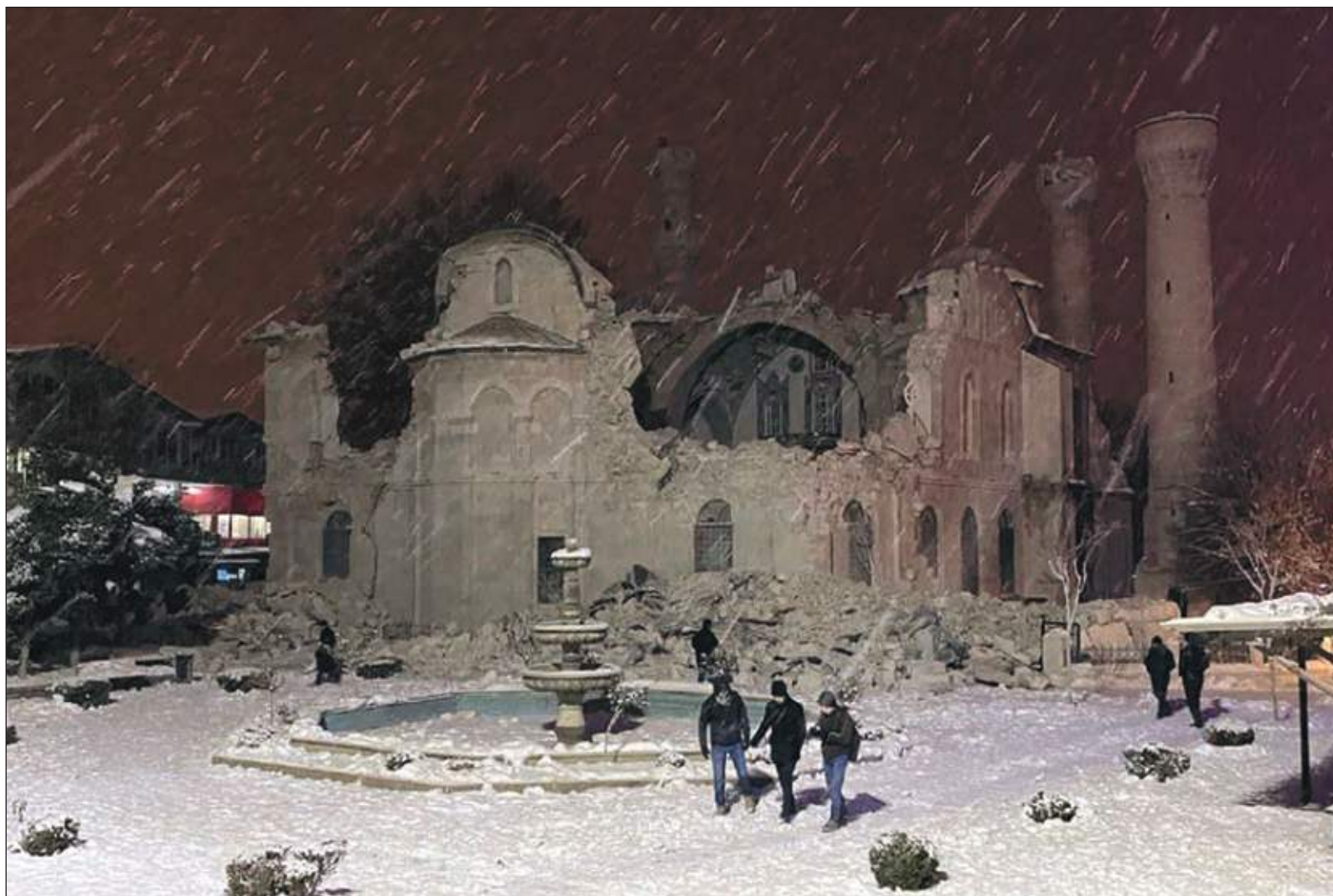
TURKEY – Damaged mosque: People walked next to a mosque destroyed by an earthquake in Malatya, Monday.
