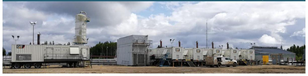
Mid-2018, Razor invested \$10 million in the design, construction and commissioning of 9 MW of natural gas reciprocating engine power generation at its South Swan Hills main battery
