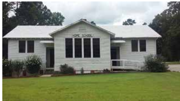
Figure 29: Hope Rosenwald School in Pomaria, Newberry County, South Carolina, before restoration (above) and after restoration (below) (SC Department of Archives & History).
