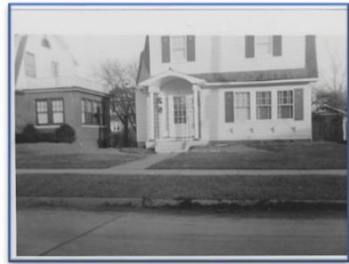
Refurbished Parsonage in August 1949
