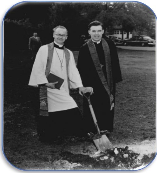
Pastors Salstrom and Gallup turn the first shovel at the ground-breaking service
