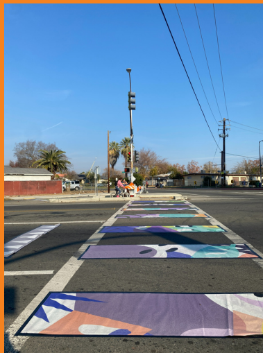
IMAGE: INSTALLED TEMPORARY CREATIVE CROSSWALK
