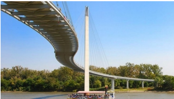
Bob Kerrey Pedestrian Bridge, Omaha, NE/Council Bluffs, IA
