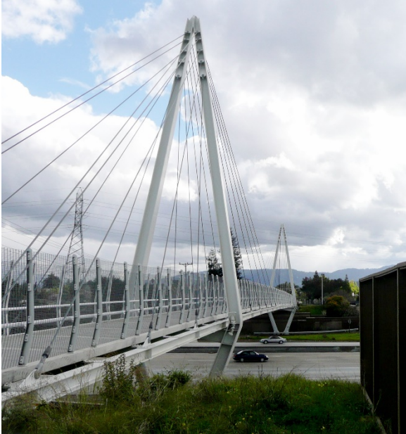
Don Burnett Bicycle-Pedestrian Bridge, Cupertino, CA
