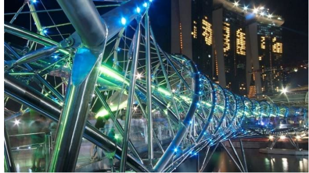
Helix Bridge. Singapore
