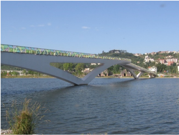
Pedro e Ines Bridge, Coimbra, Portugal
