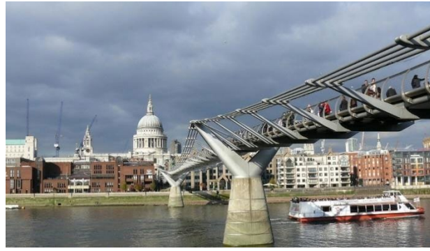
Millennium Bridge. London, UK
