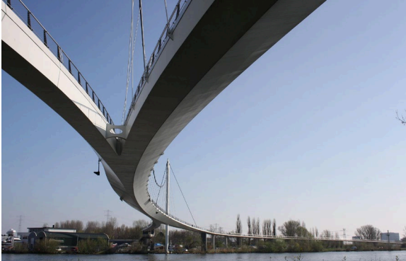
Nescio Bridge, Amsterdam, NL
