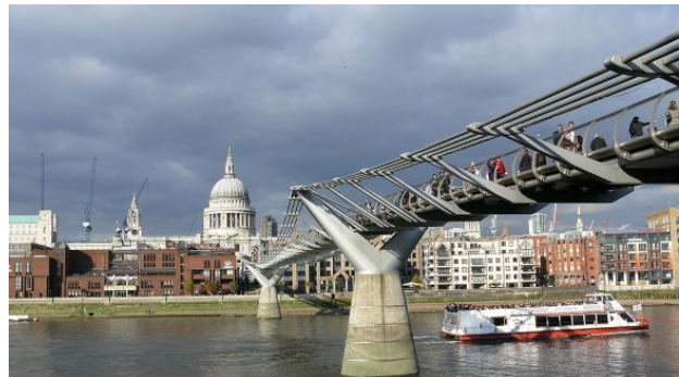
Millennium Bridge, London, UK
