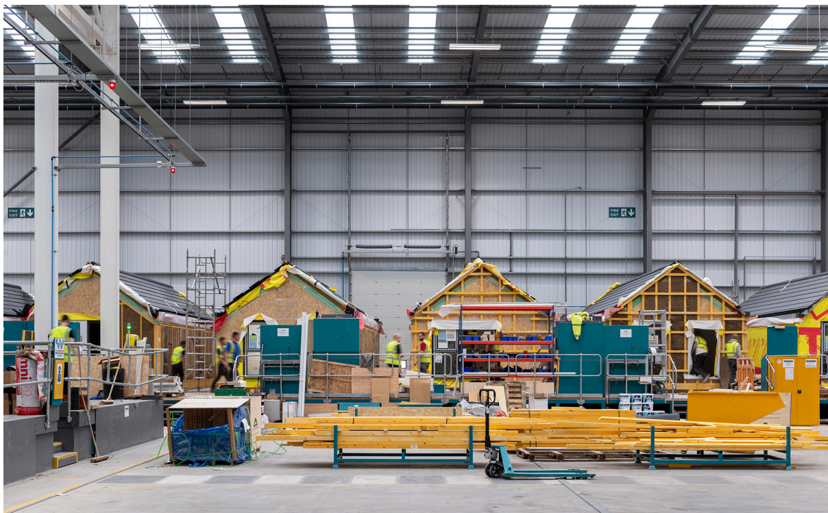
Figure 3: BoKlok homes on TopHat's factory finishing line, photo courtesy of TopHat Solutions
