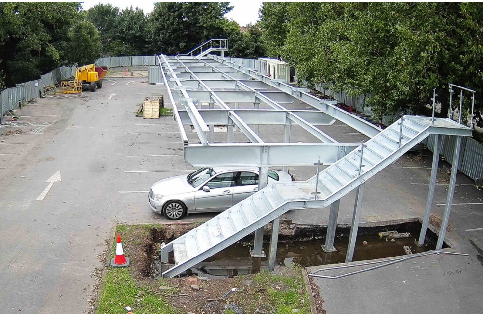
The steel framed platform structure courtesy of ZED PODS
