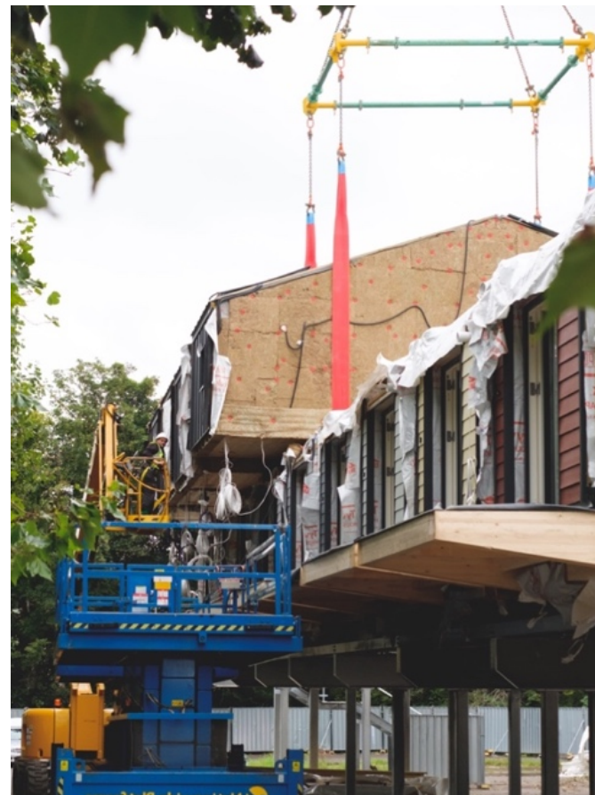
Installation of the ZED PODS, photo courtesy of @JonCraig_Photos
