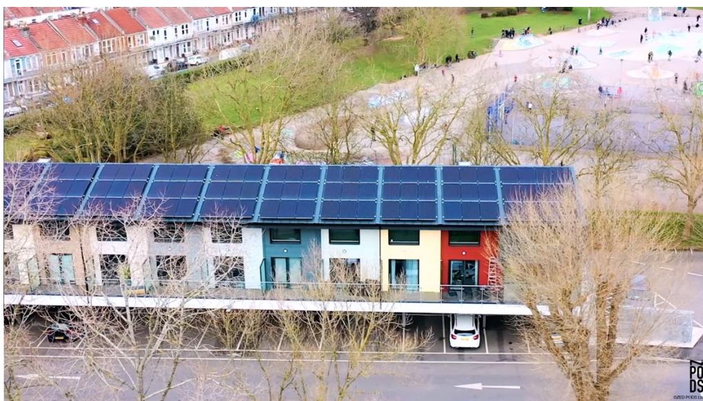
Figure 8: Hope Rise solar PV array copyright ZED PODS
