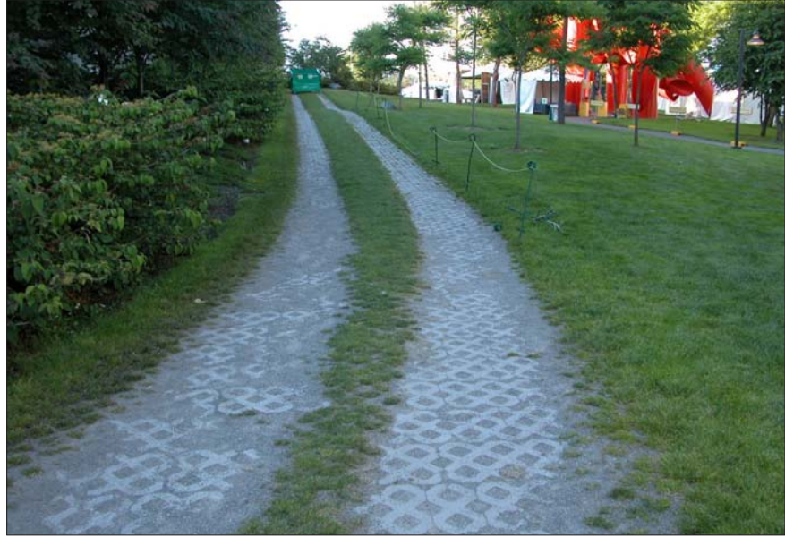
Figure 9. Surface brickwork absorbs the compressive forces of traffic and still allows some vegetation growth through voids in the brick.
