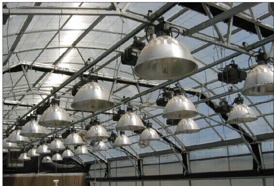
Figure 6. High intensity discharge lights can be used for supplemental lighting in a greenhouse during dark winter months.
