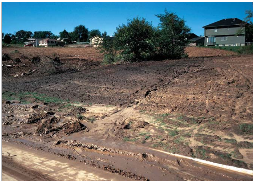
Figure 3. Uncontrolled erosion from a residential construction site. Sediment has completely filled in the street gutter. (Photo courtesy of USDA-NRCS)
