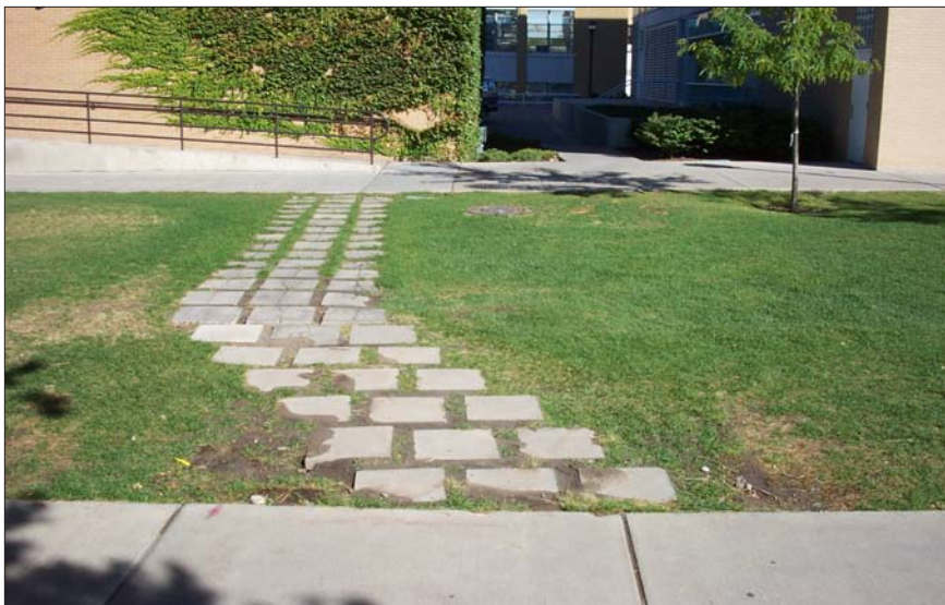
Figure 11. Surface pavers are a low-technology solution to the problem of compaction trails in turfgrass.
