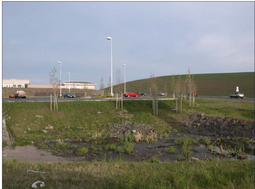
Figure 6. A stormwater catchment and infiltration basin in Pullman, Washington. These basins are now common sights in new residential and commercial developments.
