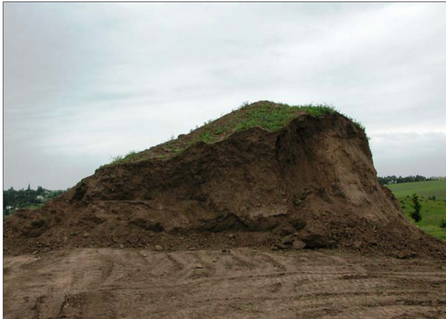
Figure 2. Soil stored in a large stockpile on a residential construction site.
