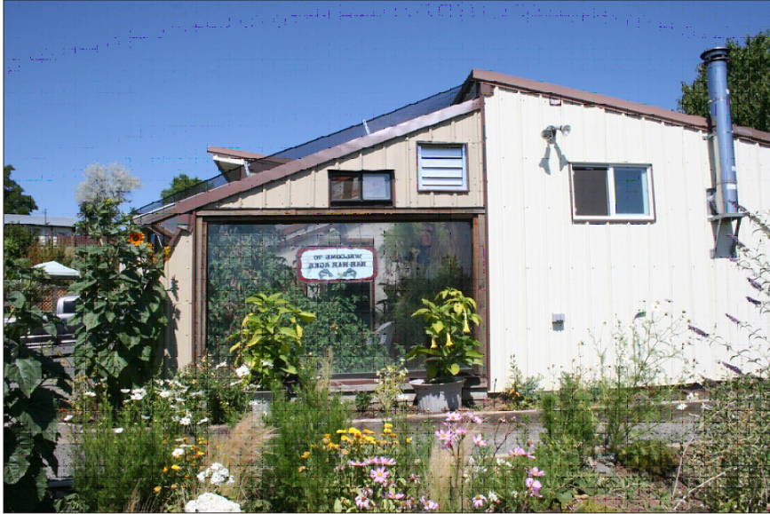
Figure 1. This lean-to hobby greenhouse is “half a greenhouse,” attached along its length to another building.
