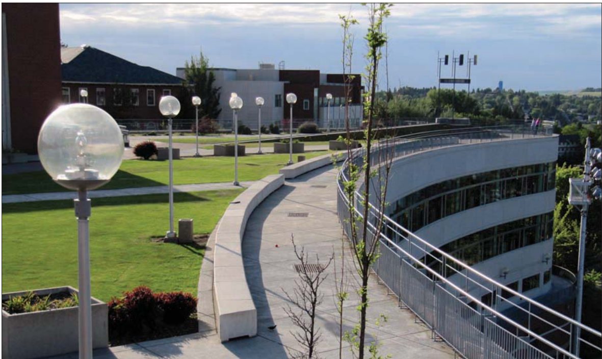
Figure 1. Turfgrass can be used as a roofing material. Here it is part of the roof of the Holland Library on the Pullman campus of Washington State University. (Photo courtesy of Gerald Steffen.)
