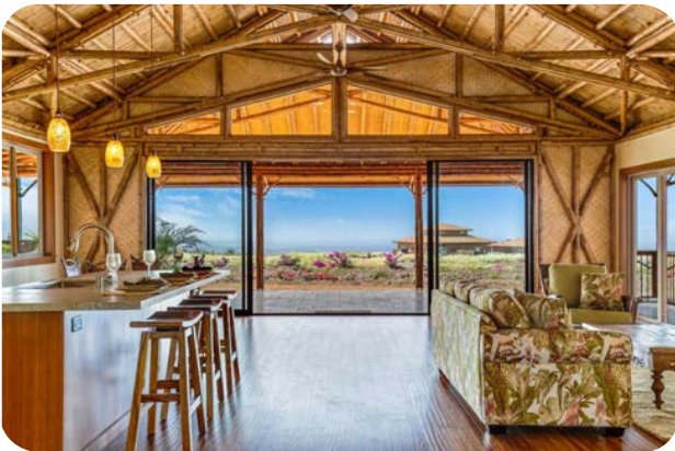
Split bamboo ceiling finish with exposed bamboo trusses.
