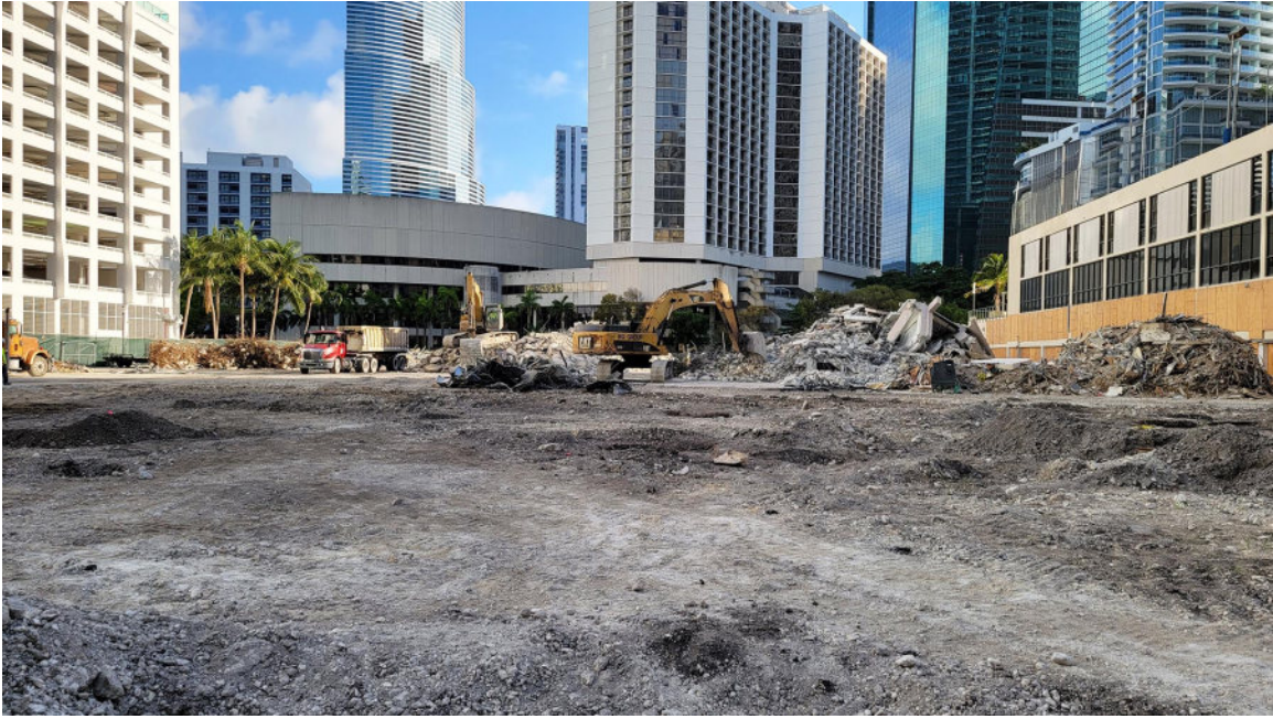
Figure 9. Project parcel looking north.
