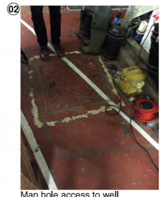
Man hole access to well
