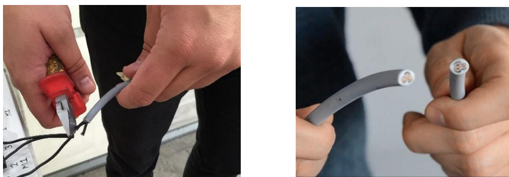
Figure 16 — Cutting power supply cable
