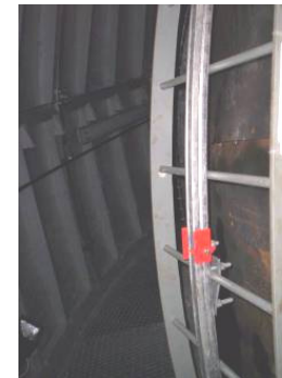
Curved rotating ladder + slide-lock eg. Glide lock fixed rail ladder climbing system
